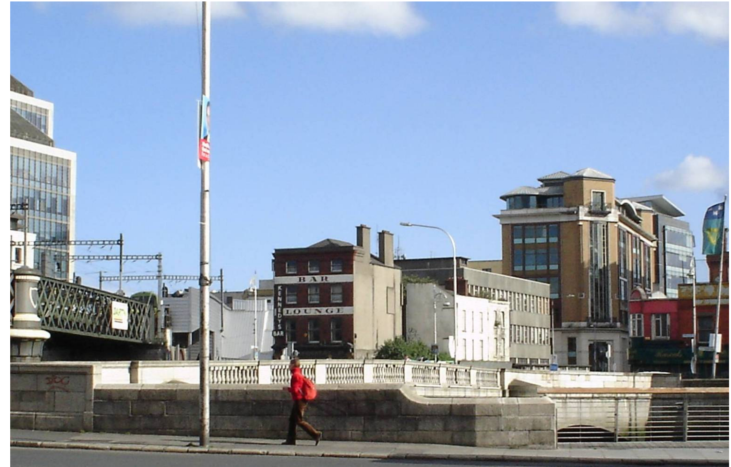
Figure 12: The Existing Site
